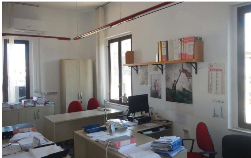
Figure 41. Third floor: recently installed window frames
