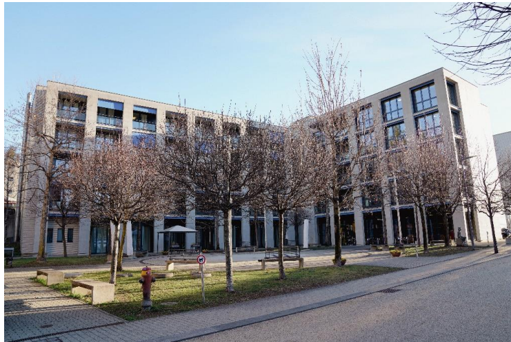
Figure 28. Casa Girasole Building
