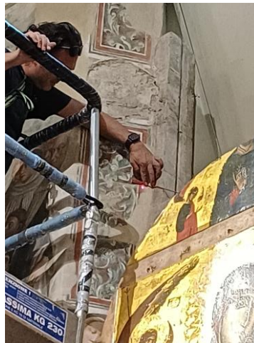
Figure 15. Installation of higher sensors next to the window
