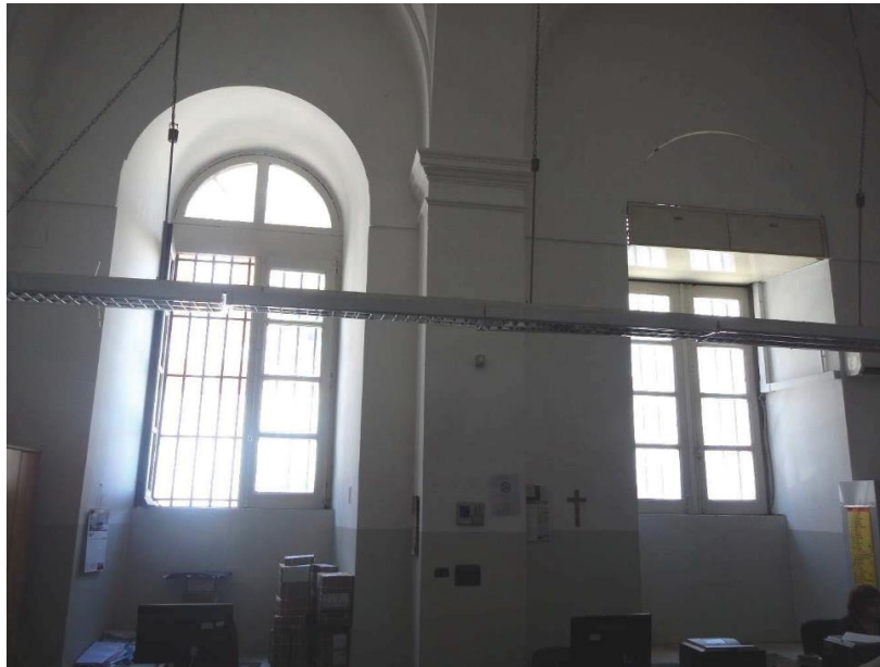
Figure 40. Ground floor: large openings in the west wing of the building
